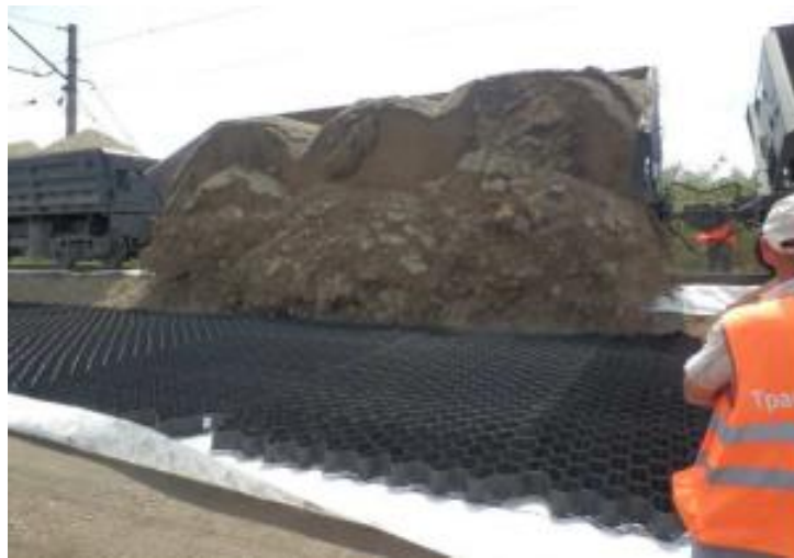
Figure 2.9 Geocell-Geotextile Hybrid System
