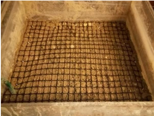
Figure 3.27 Geogrid Installation in HGRS Section
