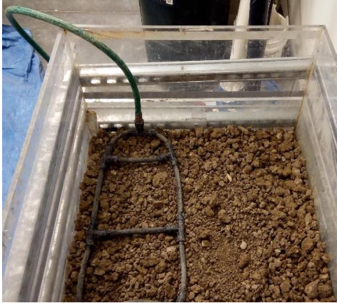
Figure 3.15 Placement of Soaker System at the Top Half of Subgrade
