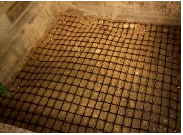
Figure 3.23 Geogrid Placement
