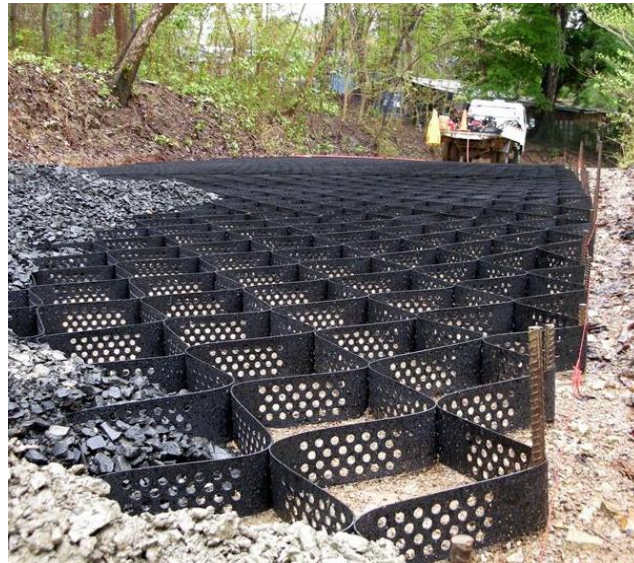
Figure 2.5 Geocell Application in Roadway
