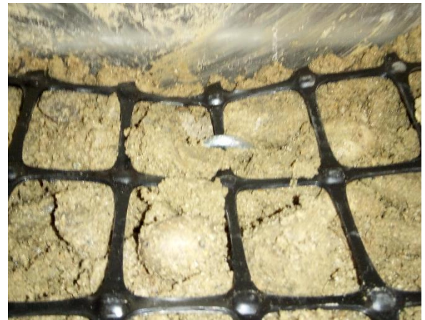
Figure 3.25 Anchoring Geogrid using Steel Peg
